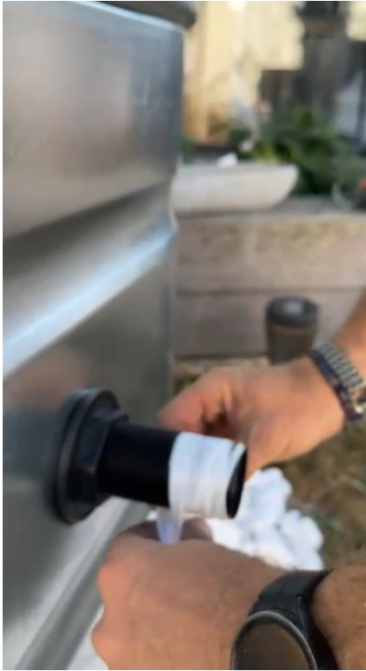
Wrap the male thread with PTFE tape.
