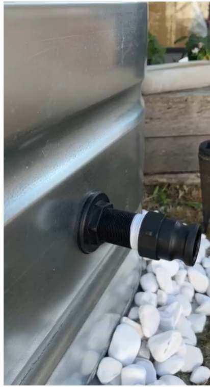
Screw the adaptor into the fitting.
