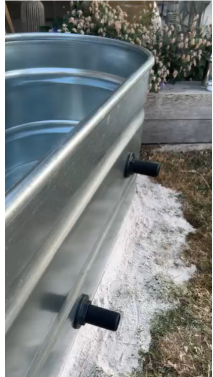
Both outlets installed and aligned.
