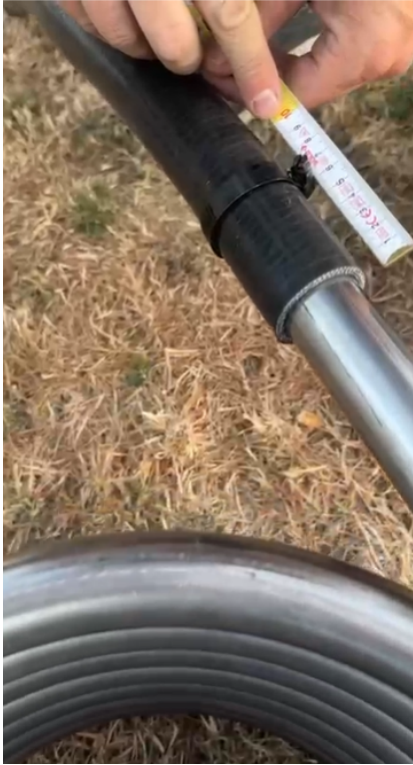
Measure the required hose length.
