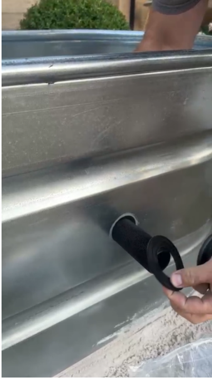
Insert and tighten the first fitting.
